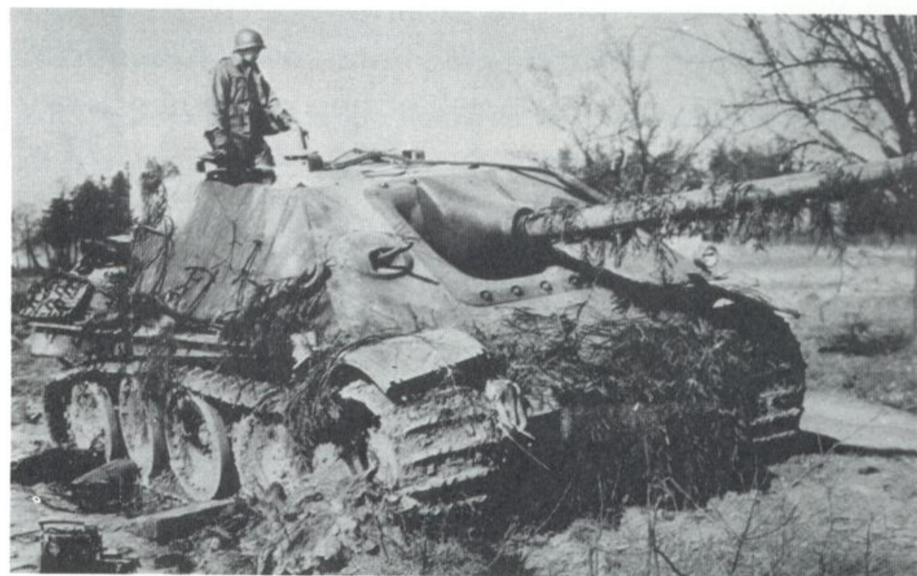
Along with two-piece barrels, single-piece barrels were also used on the Jagdpanther. This one also carries the bolted collar.
