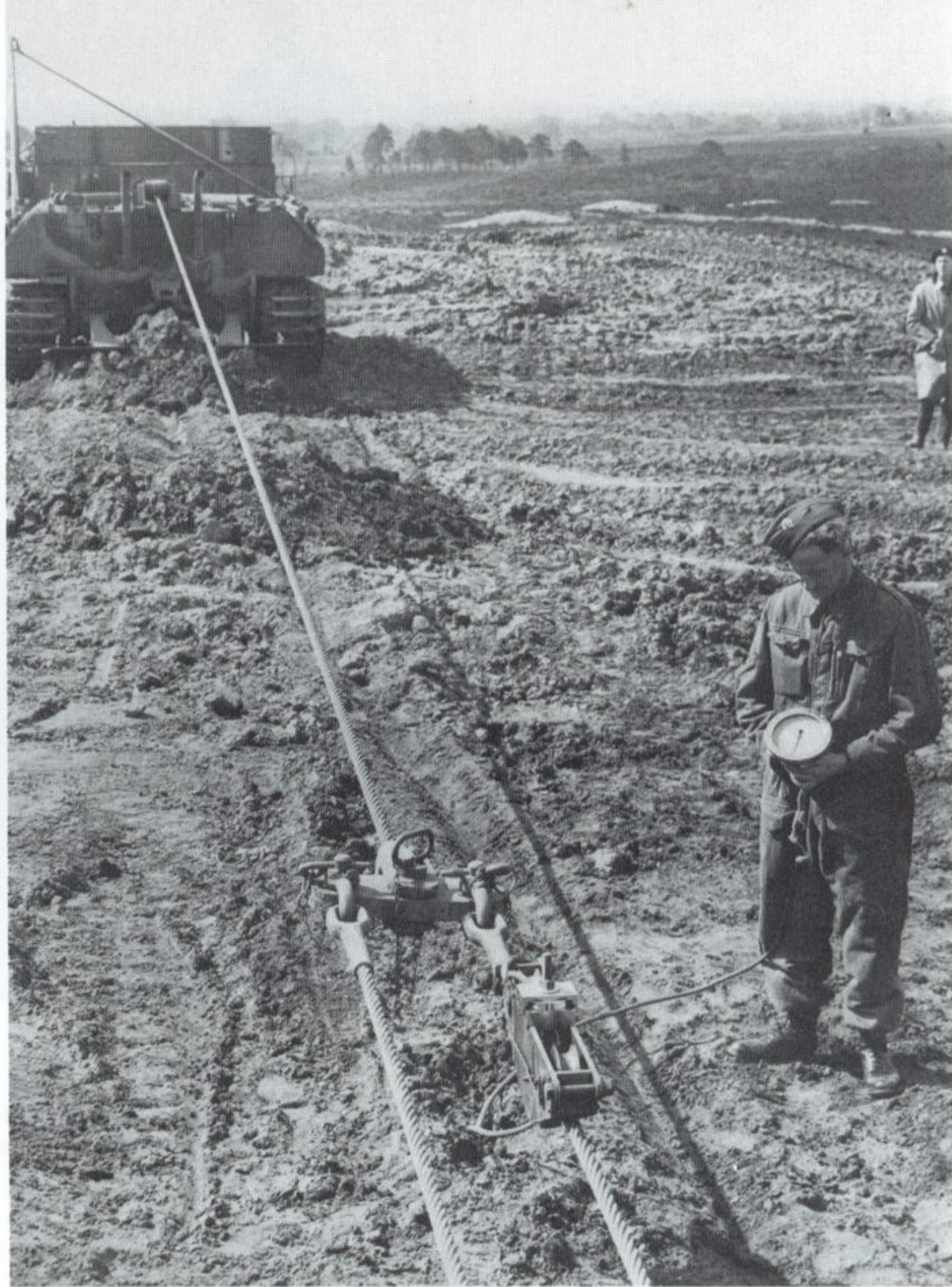
British forces gauging the pulling power of a Bergepanther.
