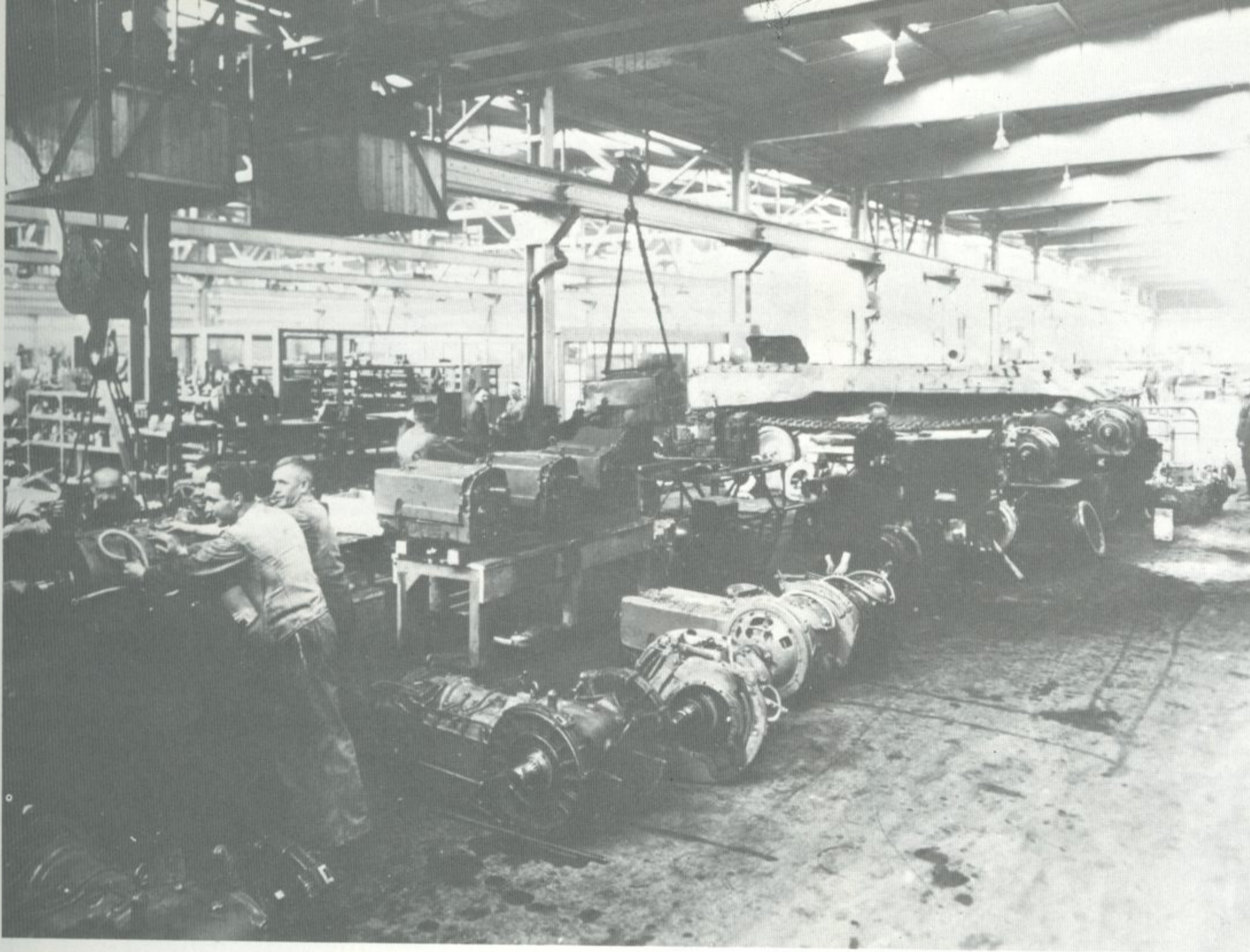
The finished chassis is lowered onto the tracks.
