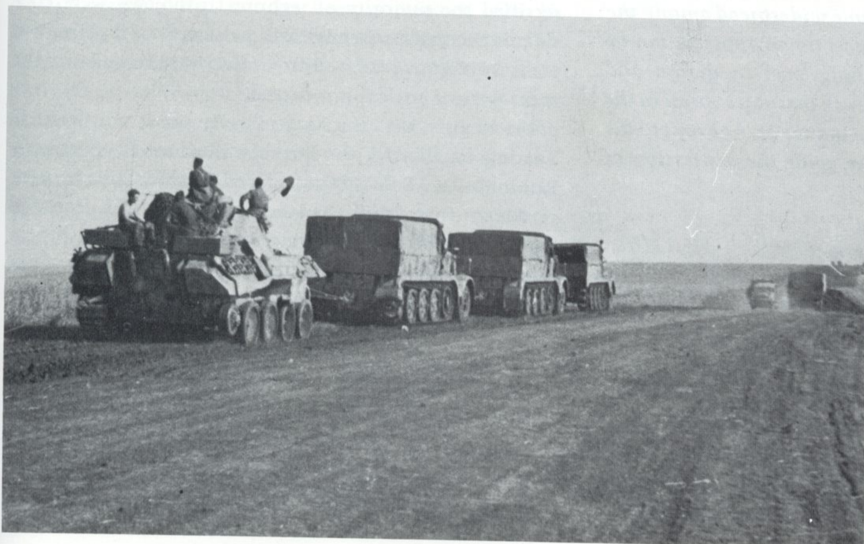
The 18 ton half-tracks were only able to recover damaged vehicles in a train of three.
