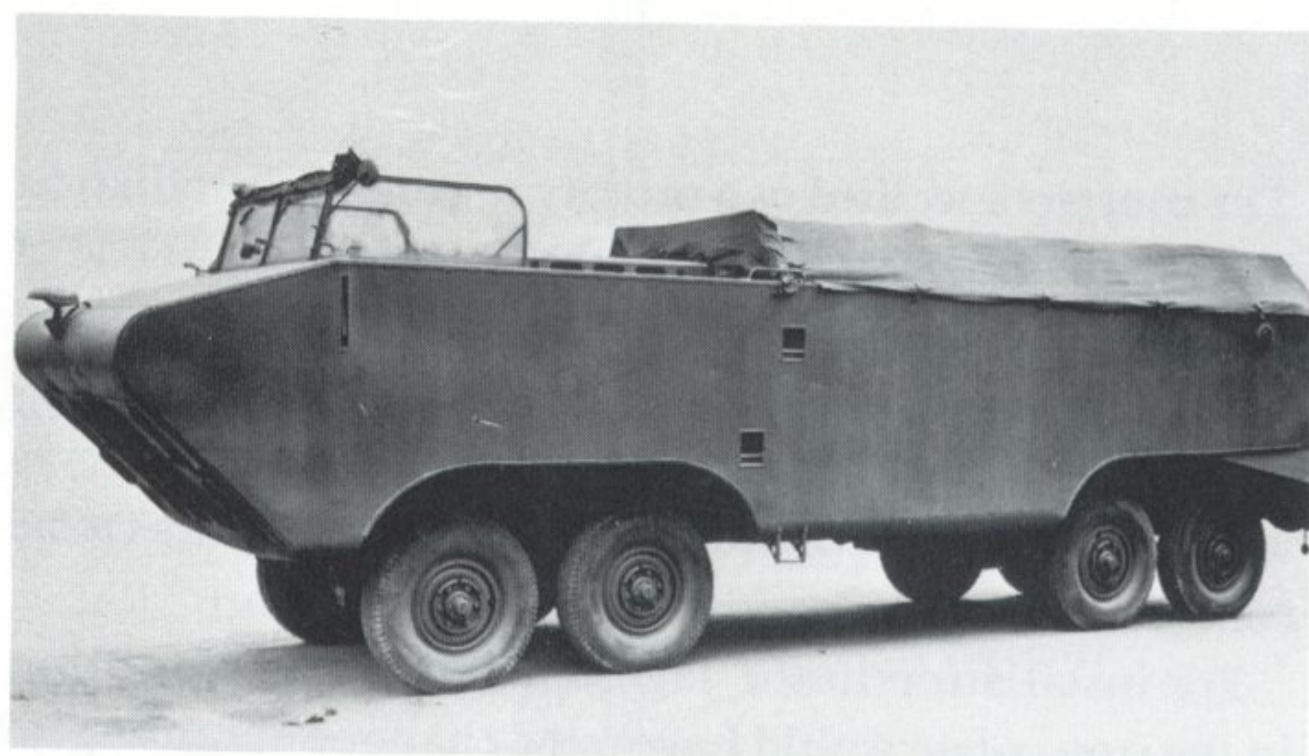
The Pionier-Sonderfahrzeug (specialized engineering vehicle) developed by Maschinenfabrik Augsburg-Nürnberg was designed as an amphibious vehicle for creating obstacles and was to tow a heavy trench-forming plow.
