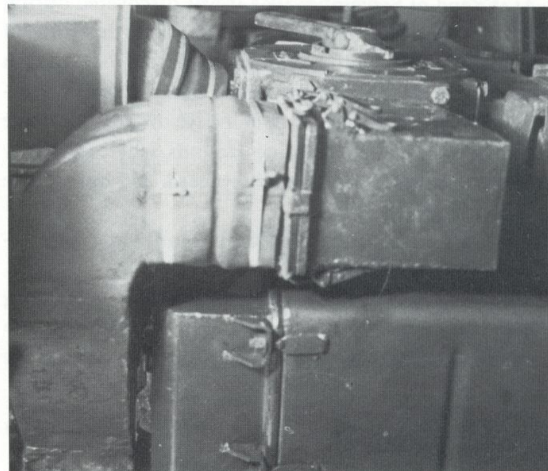
Pre-filter box with blower intake for the air filtration system.
