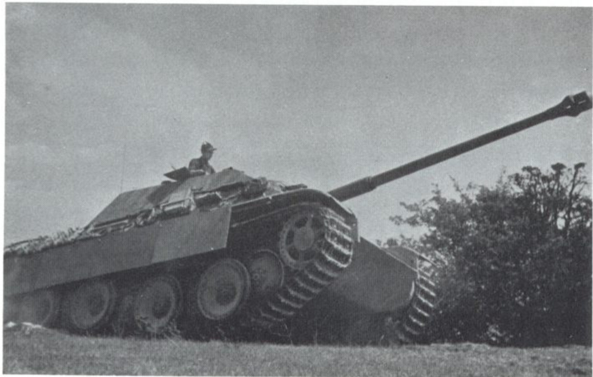
The running gear was not changed from the Panther tank.
